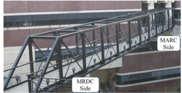
Fig. 4. Picture of the space frame bridge on the Georgia Tech campus.
