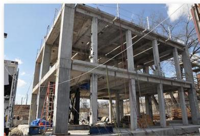
Georgia Tech test structure, designed using the 1963 ACI-318. Design parameters and details did not consider seismic loading, which is typical of older RC construction in the central and eastern US.
